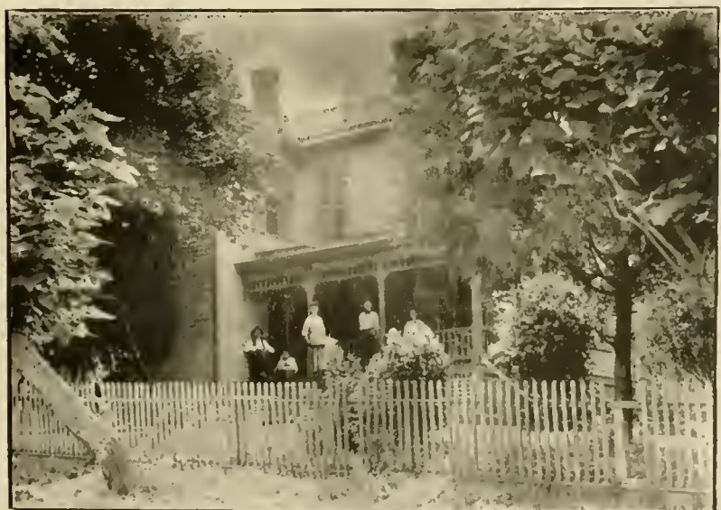
RESIDENCE OF HENRY A. BINGAMAN. South 7th Street.
